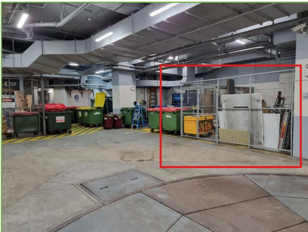
Figure 6: Chain-link fencing along eastern side of loading dock shown by red rectangle
